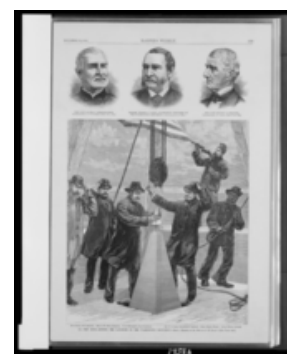
P. H. McLaughlin setting the aluminum apex with Thomas Lincoln Casey (hands up)
