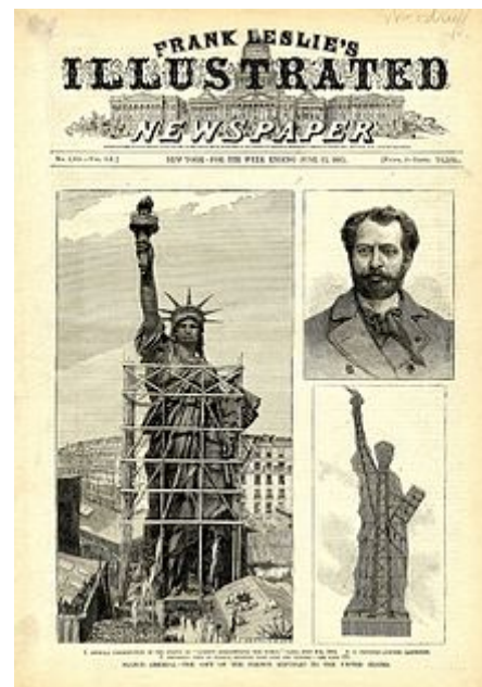
Frank Leslie's Illustrated Newspaper , June 1885, showing (clockwise from left) woodcuts of the completed statue in Paris, Bartholdi, and the statue's interior structure
