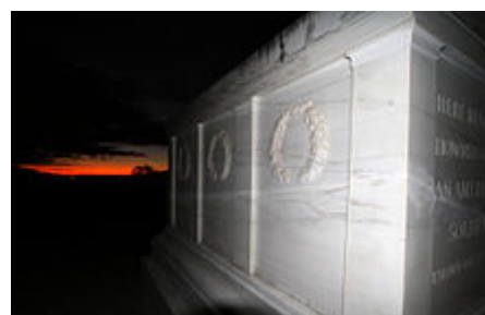
October 21, 2011: Completed repair of the cracks in the Tomb.
