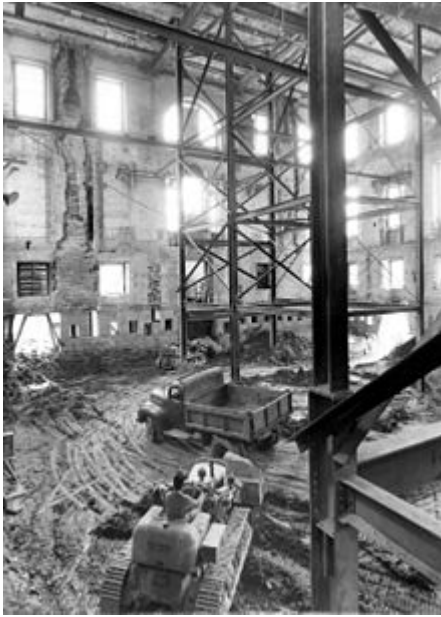
Truman reconstruction, 1949–1952. A steel structure is built within the exterior shell.
