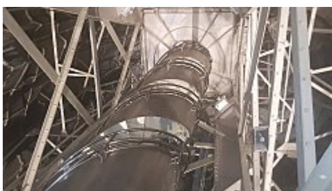
The new staircase to the crown
