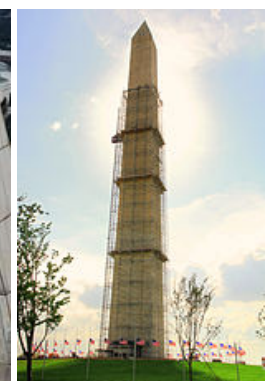
Repairs on the Washington Monument in 2013
