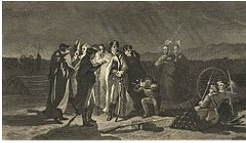
Lieutenant Colonel Washington holds night council at Fort Necessity
