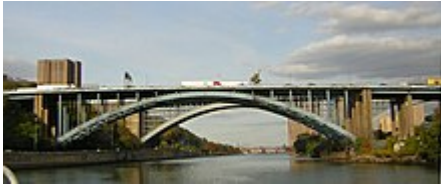
A view of the Alexander Hamilton Bridge from the south
